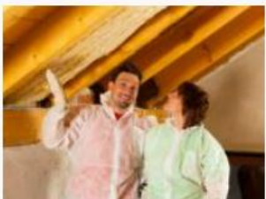
Attic Air Sealing
